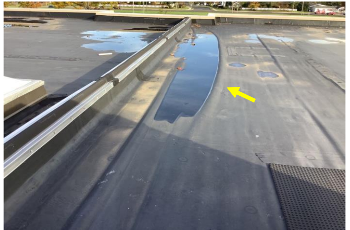
Defect 4 – View of wrinkles found along the North perimeter of Roof Area C. There is approximately (40 LFT.) forty linear feet of wrinkles were noted at time of inspection.
