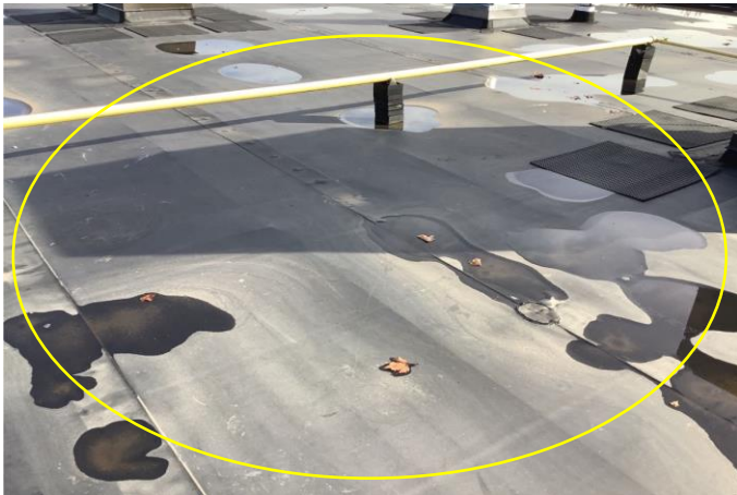
Defect 7 – Overview of ridging and buckling insulation near the South perimeter of Roof Area C. There was approximately (1,450 SQFT.) one thousand four hundred fifty square feet of buckling insulation documented at time of inspection.
