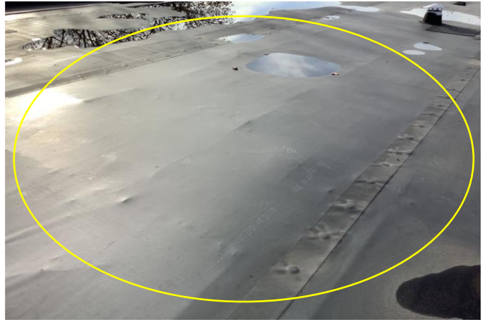
Defect 6 – Another view of ridging and buckling insulation near the South perimeter of Roof Area C.
