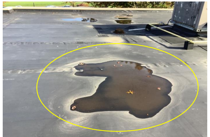
Defect 11 – Another View of ponding water found near the North perimeter of Roof Area A. Approximately (440 SQFT.) four hundred forty square feet of ponding water was noted at time of inspection.
