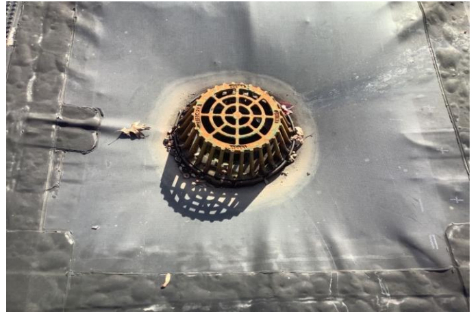
6 - Drain (Internal). Count: 10
