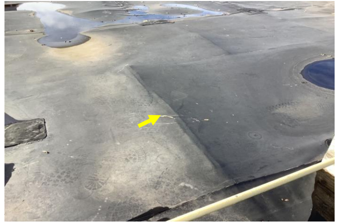
Defect 2 - View of buckling insulation found near the West perimeter of Roof Area B.
