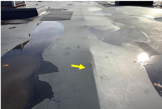
Defect 2 – Another view of buckling and ridging insulation found near the West perimeter of Roof Area B.
