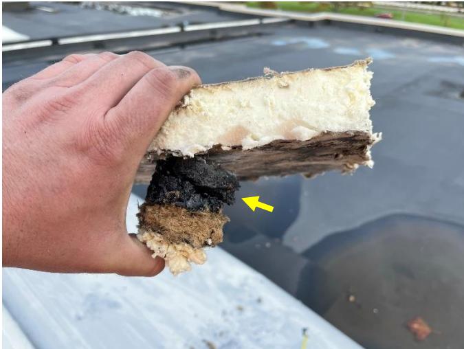
View of core-cut taken on Roof Area B. The single-ply roofing system consists of a mechanically attached EPDM membrane with 1.50" of polyisocyanurate. No moisture was documented at core-cut location. Picture #7
