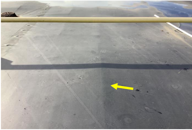
Defect 5 - View of ridging insulation found near the West perimeter of Roof Area C.
