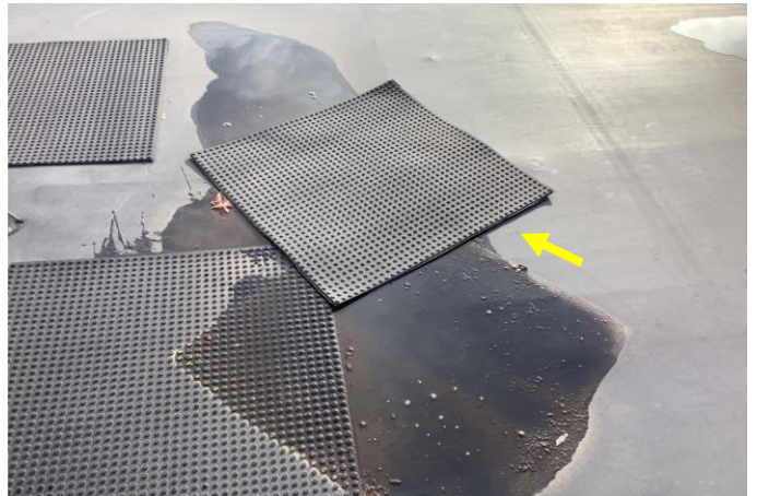
Defect 18 – View of an unsecured walk pad found near the East perimeter of Roof Area C. There was (1) one unsecured walk pad noted at time of inspection.
