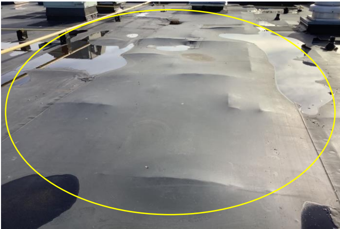
Defect 11 – Another view of ridging insulation near the South perimeter of Roof Area B.
