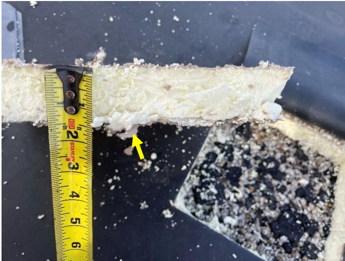
View of core-cut taken on Roof Area A. The single-ply roofing system consists of a mechanically attached EPDM membrane with 1.50" of polyisocyanurate. No moisture was documented at core-cut location. Picture #7
