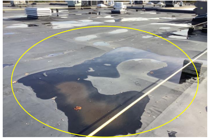
Defect 4 - View of ponding water found near the West perimeter of Roof Area B.
