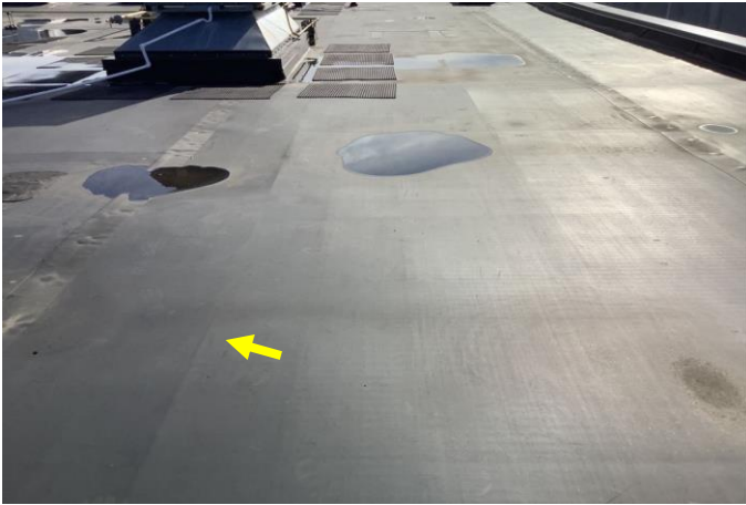
Defect 1 – View of minor ridging insulation found near the North perimeter of Roof Area A. Approximately (50 SQFT.) fifty square feet of minor ridging insulation was noted at time of inspection.
