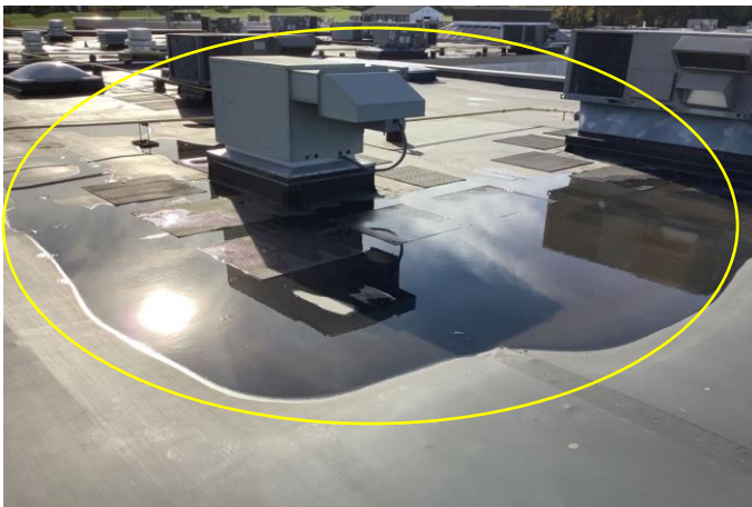
Defect 10 – View of ponding water found near the West perimeter of Roof Area A. Monitor membrane at ponding water for early membrane deterioration.
