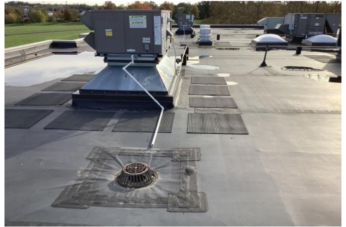
Overview of the drainage system on Roof Area C. The drainage consists of interior drains near the perimeter of the roofing system. Picture #4
