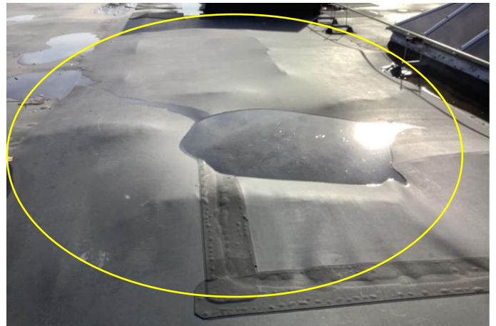
Defect 2 - Another view of buckling insulation found near the West perimeter of Roof Area B.
