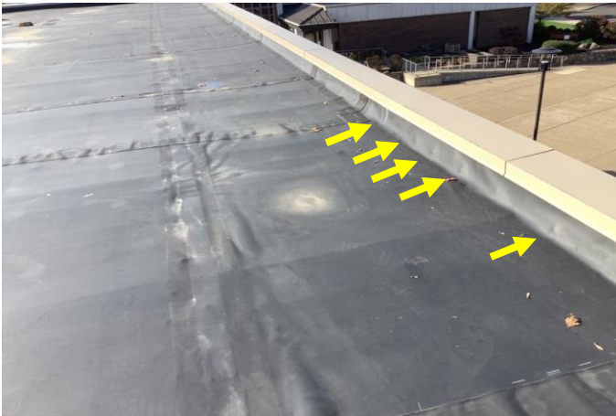
Defect 3 – Overview of backing out fasteners at the North perimeter of Roof Area A. Approximately (24) twenty-four backing out fasteners were noted at time of inspection.
