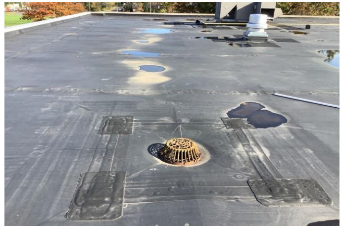
Overview of the drainage system on Roof Area A. The drainage consists of interior drains near the perimeter of the roofing system. Picture #6
