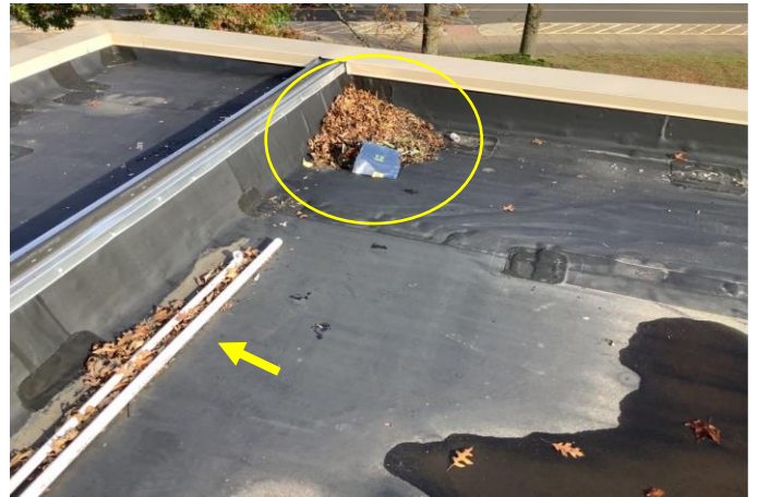
Defect 13 – View of debris and broken condensation lines found along the North perimeter of Roof Area B. Clear all debris from roof to allow for proper drainage of the roofing system. Approximately (6 SQFT.) six square feet of debris was noted at time of inspection.
