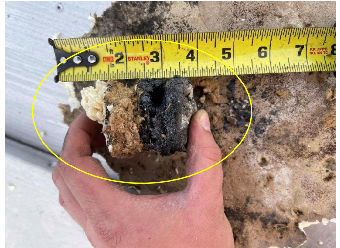
View of core-cut taken on Roof Area B. The roof consists of a mechanically attached EPDM roof, 1.50" polyisocyanurate insulation, gravel asphalt built-up roof, 1.00" wood fiber board, 1.50" polyisocyanurate insulation and a steel deck. Picture #8
