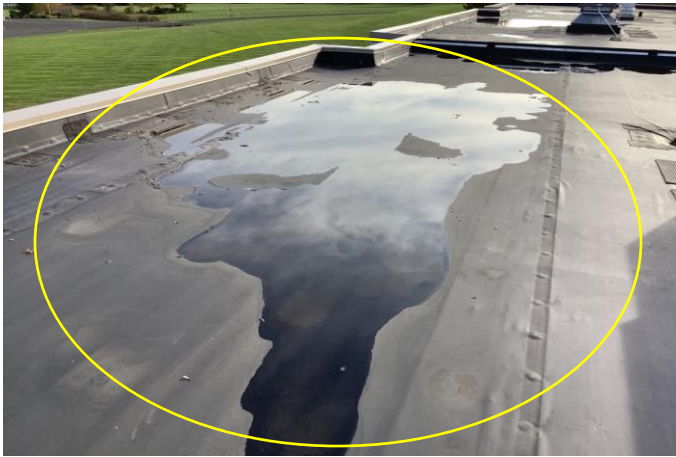
Defect 16 – Overview of ponding water found along the East perimeter of Roof Area B. Approximately (1,800 SQFT.) one thousand eight hundred square feet of ponding water was documented at time of inspection.
