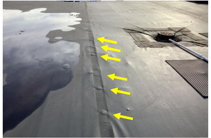
Defect 15 – Overview of backing out fasteners found near the East perimeter of Roof Area B. There were approximately (150) one hundred fifty backing out fasteners documented at time of inspection.
