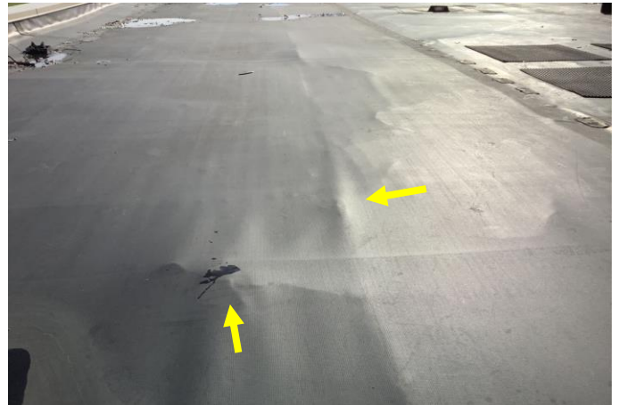
Defect 4 – View of buckling insulation found near the East perimeter of Roof Area A.
