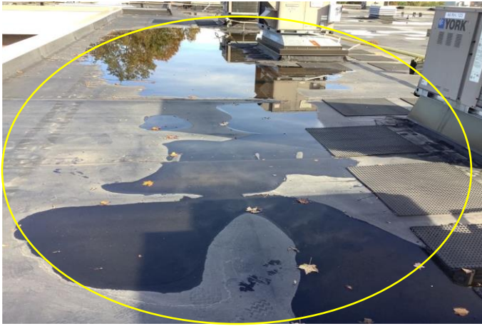
Defect 1 - View of ponding water found along the North perimeter of Roof Area B. Monitor membrane at ponding water for early membrane deterioration.
