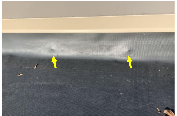
Defect 3 – View of backing out fasteners along the North perimeter of Roof Area A.
