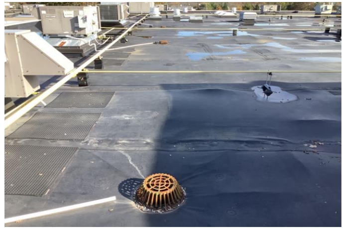
Overview of the drainage system on Roof Area B. The drainage consists of interior drains near the perimeter of the roofing system. Picture #6
