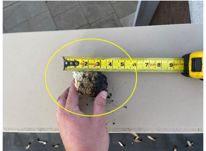
View of core-cut taken on Roof Area A. The roof consists of a mechanically attached EPDM roof, 1.50" polyisocyanurate insulation, gravel asphalt built-up roof, 0.75" wood fiber board, 6.0" polyisocyanurate insulation and a steel deck. Picture #8
