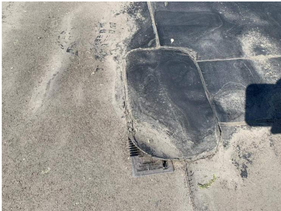
Photo #10 – Failed patch located in ponding area
