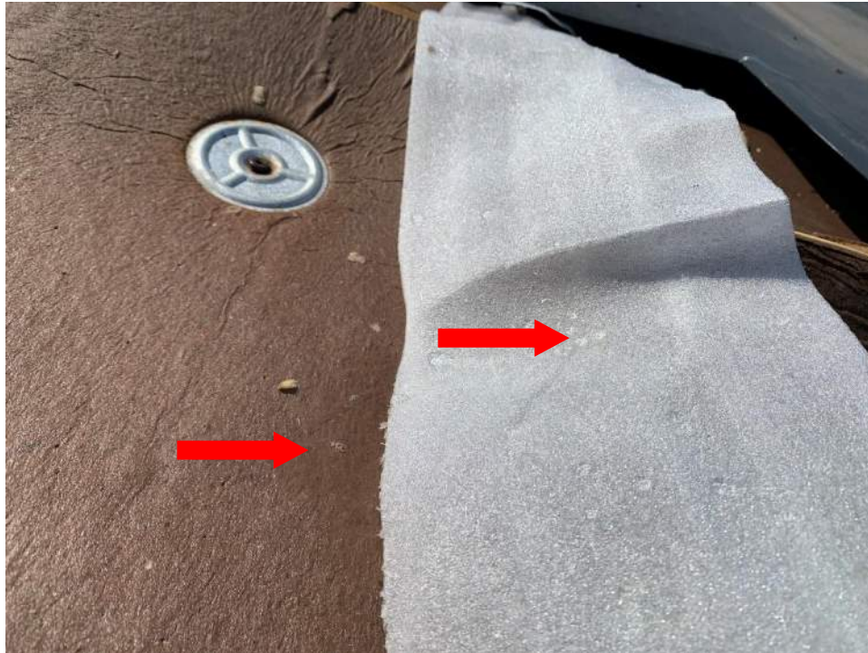
Photo #19 – Moisture underneath EPDM and on Styrofoam strip from the EPDM roll at Invasive Location #2
