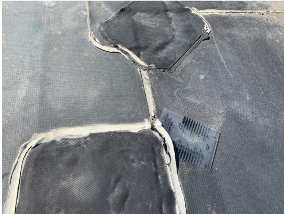
Photo #11 – Failed patch
