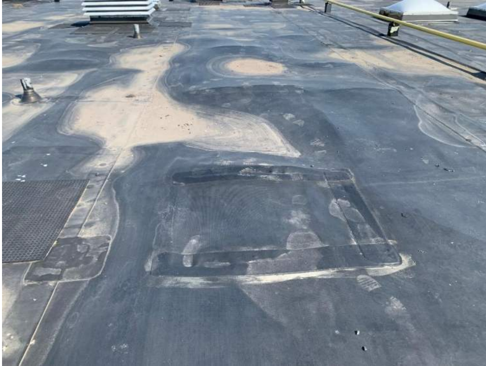
Photo #3 – Warped and displaced insulation underneath membrane
