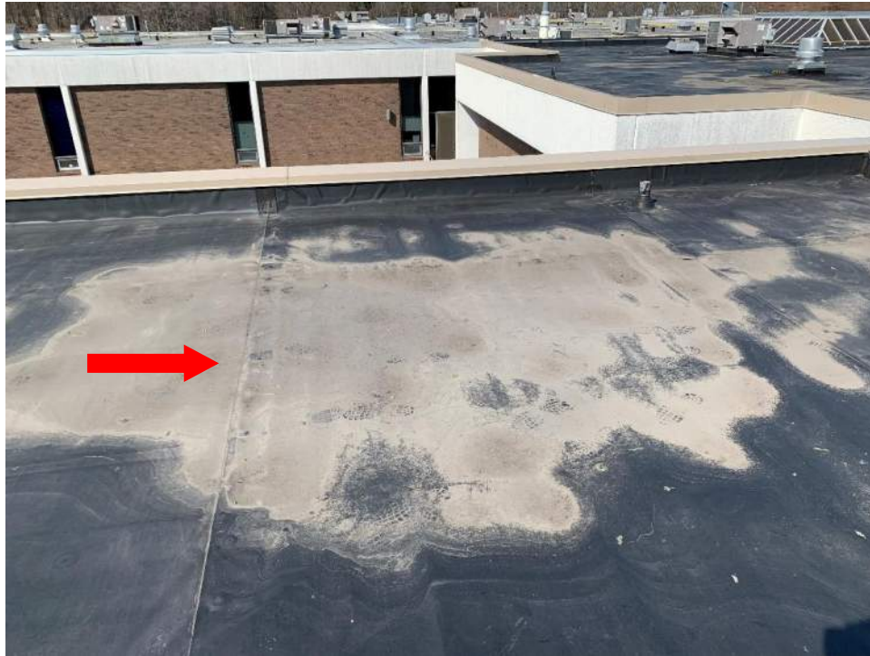
Photo #7 – Evidence of long-term ponding
