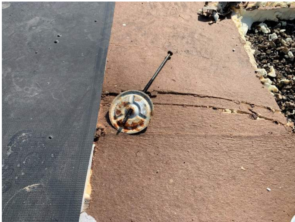
Photo #22 – Rusting plates on fasteners
