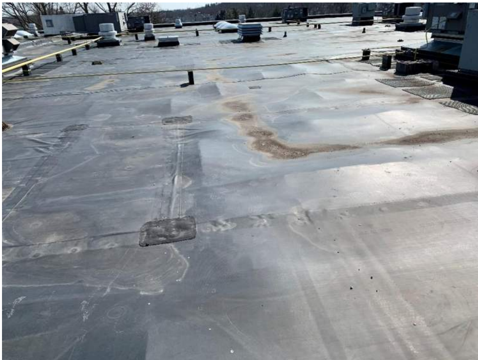
Photo #4 – Warped and displaced insulation underneath membrane
