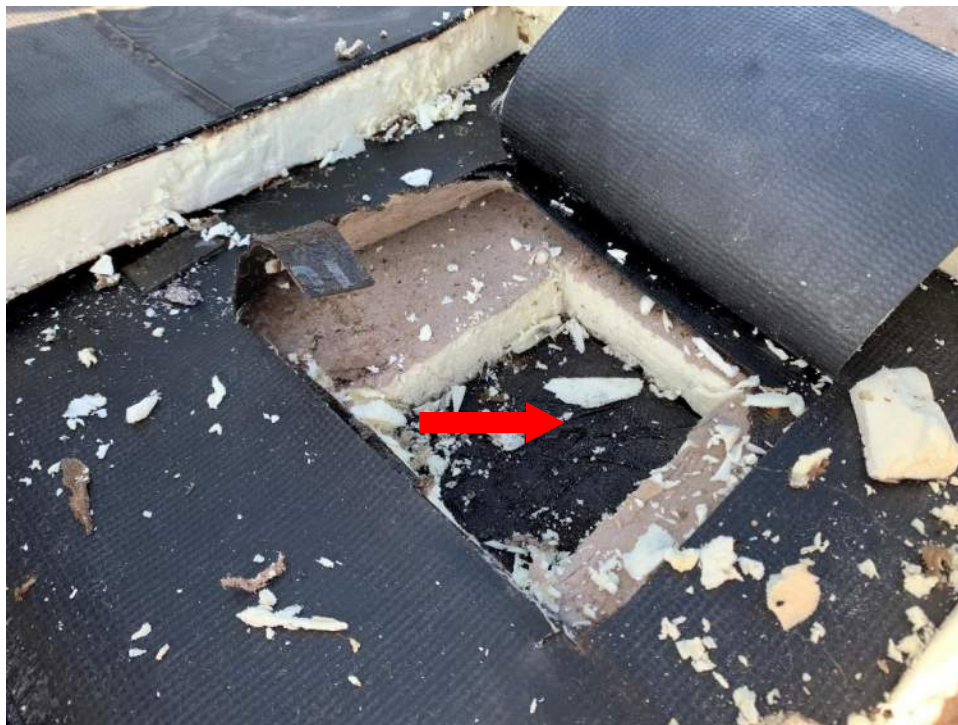
Photo #18 – Built-up roofing with gravel removed
