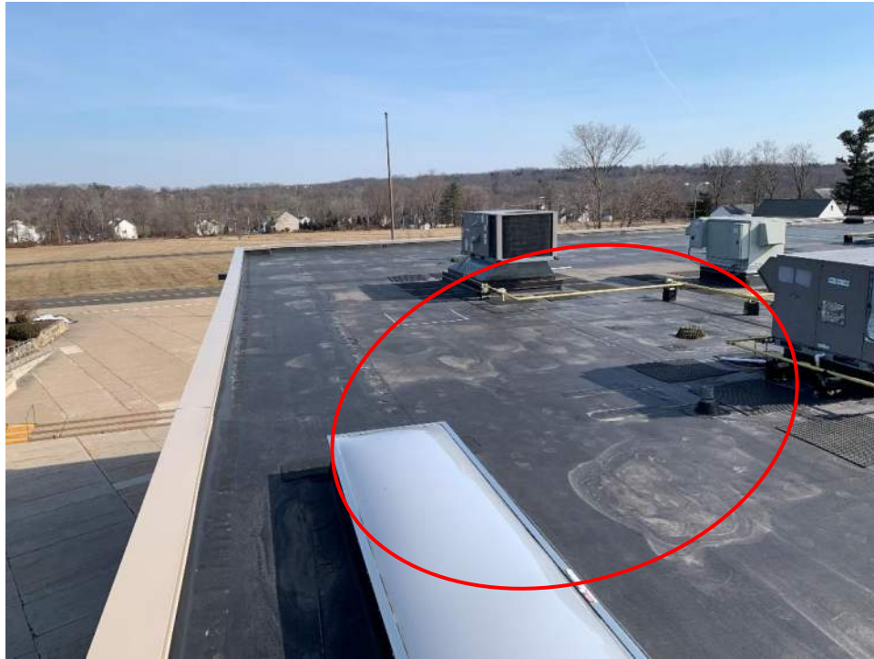
Photo #13 – Metal coping in good condition and flat insulation toward rear (oval)
