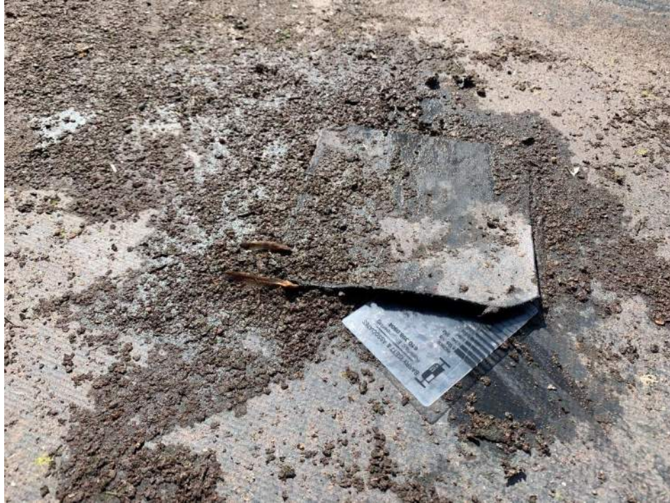
Photo #9 – Failed patch located in ponding area
