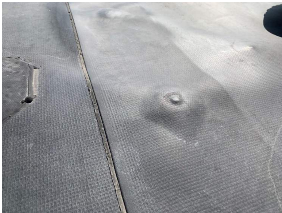
Photo #12 – Protruding fastener underneath membrane
