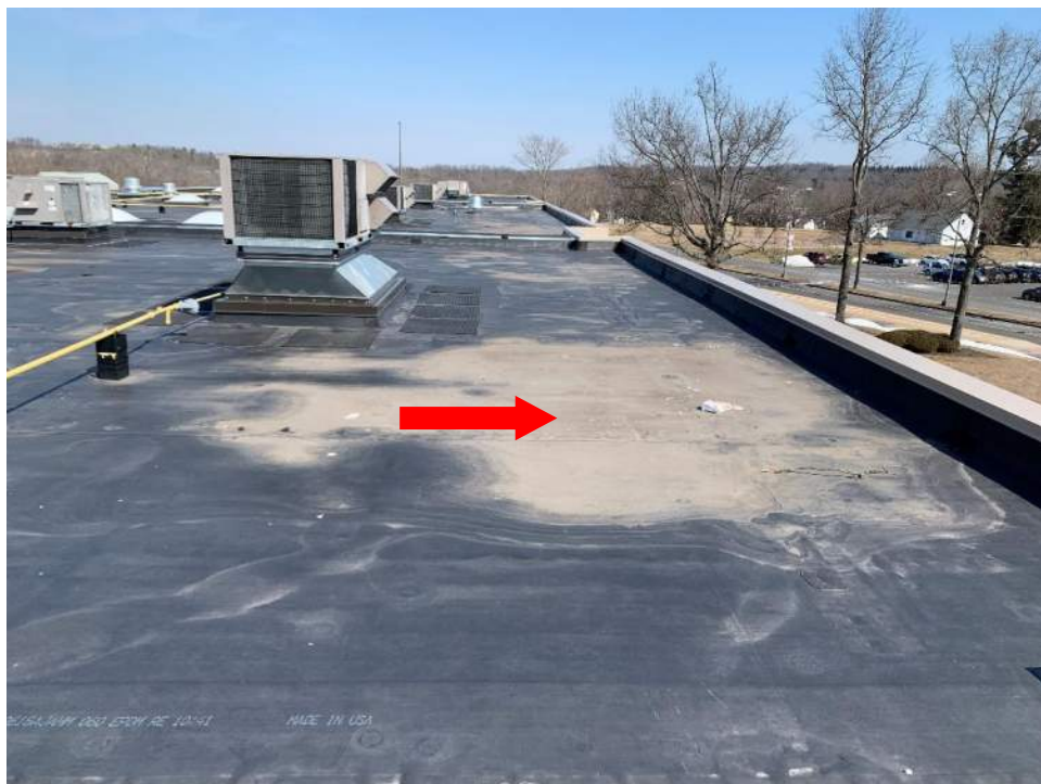
Photo #8 – Evidence of long-term ponding
