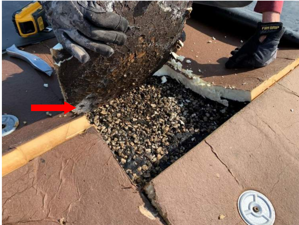
Photo #21 – Organic growth (arrow) and loose gravel at Invasive Location #2
